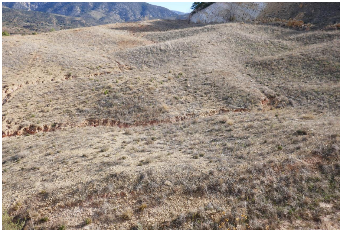
Figure 1. Panoramic view of Eastern GeoFluv (=Conventional GeoFluv without tree holes) in 06.12.2023. No rill system has developed and vegetation is not limited by erosion. The photo above is of the western side and the photo below is of the eastern side.
