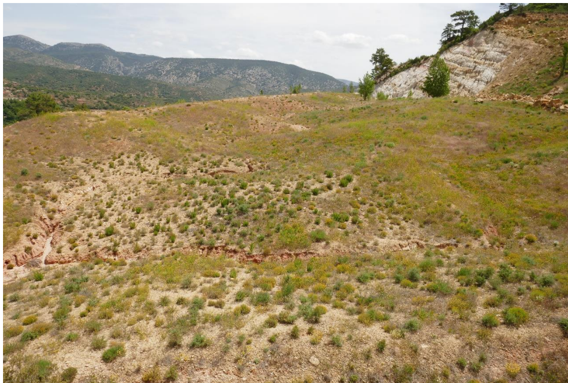
Figure 1. Panoramic view of Eastern GeoFluv (=Conventional GeoFluv without tree holes) in 05.06.2025. No rill system has developed and vegetation is not limited by erosion. The photo above is of the western side and the photo below is of the eastern side.
