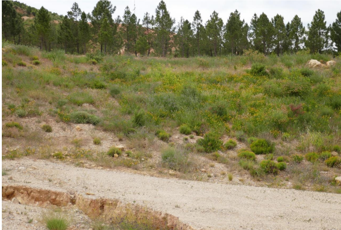
Figure 4. Western GeoFluv, the restored zone with overburden substrate. There is no difference in the number and size of the rills between the top photograph (February 2022) and the intermediate photograph (December 2023), which indicates a stabilisation of the erosive forms. Rills density in 2022 was about 0.32 \text{ m/m}^2 , below the 0.60\text{-}0.70 \text{ m/m}^2 that is considered the threshold above which erosion prevents vegetation development in restored mining areas very similar to Fortuna quarry (Moreno de las Heras et al., 2009; 2011). Observations made in June 2025 (photograph below) shows higher plant cover due to the mild spring time.
