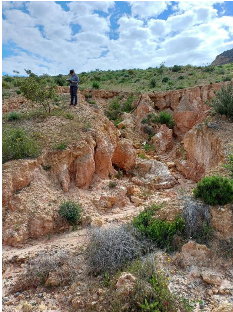
Figure S10. Big gully developed in the RU-1 because of flow concentration from upper parts of this unit. This highlights the relevance of creating a good geomorphological design avoiding steep slopes and promoting materials and textures in the soil surface to favor soil infiltration.
