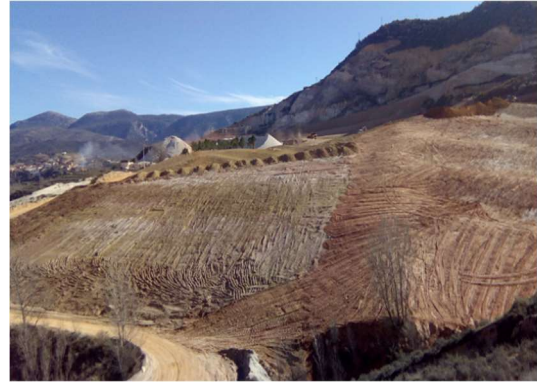
Photo 25. Application of the colluvion.
