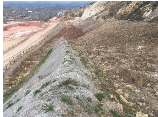
Photo 23. Rough and loose technical.
