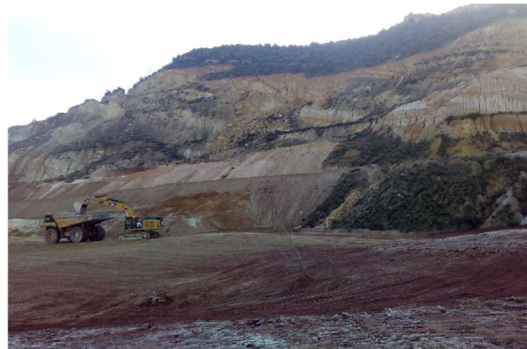
Photo 21. GeoFluv model construction.
