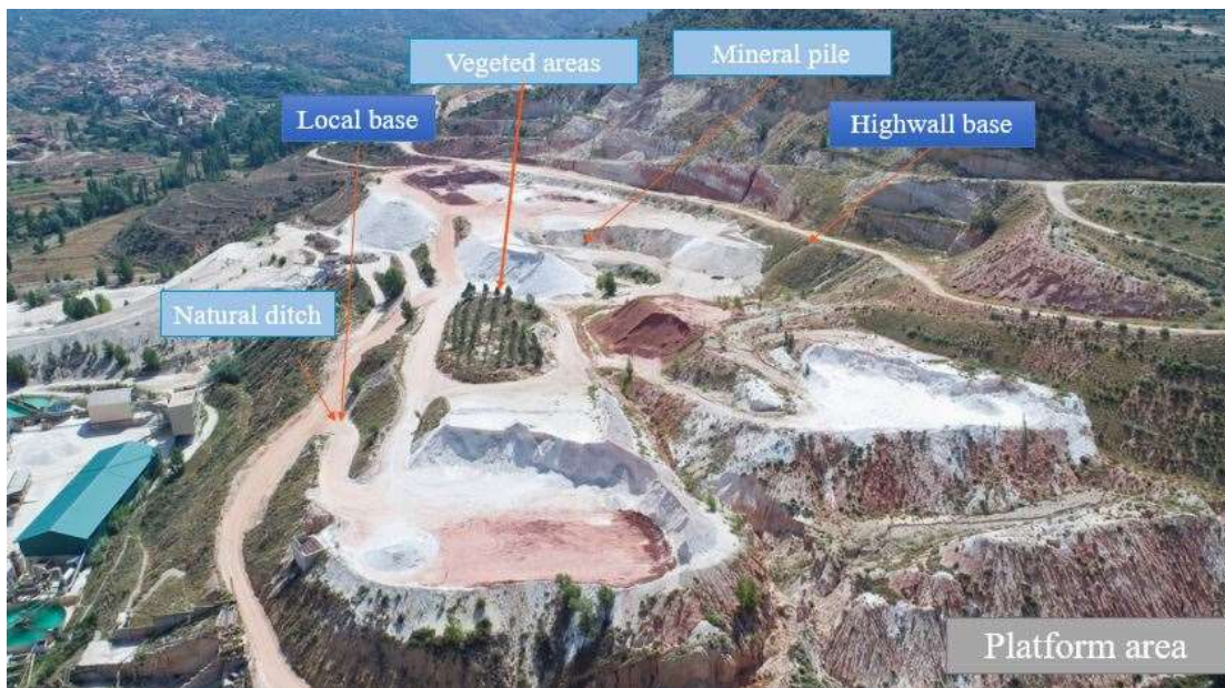
Platform area (Aerial photograph). June 2018
