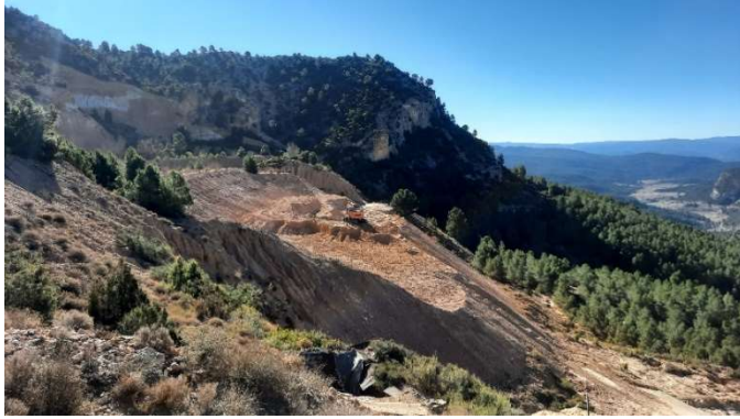
Figure 2 Cabezo-bis mine during works
