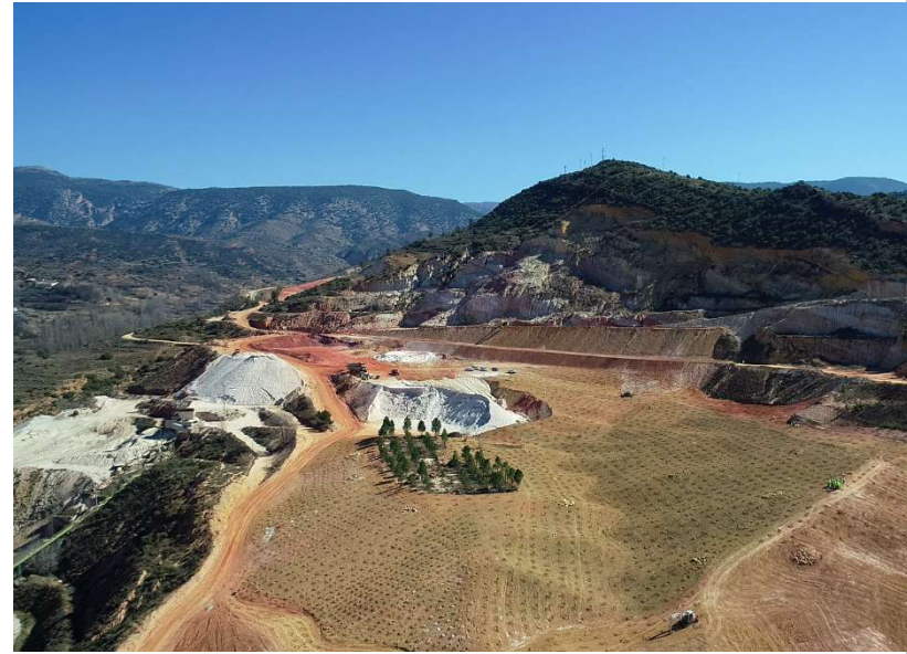
Platform area after. April 2019
