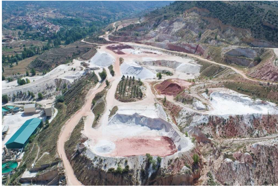
Platform area before. June 2018
