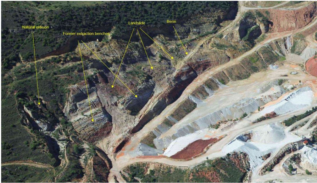
Starting point of the slope area
