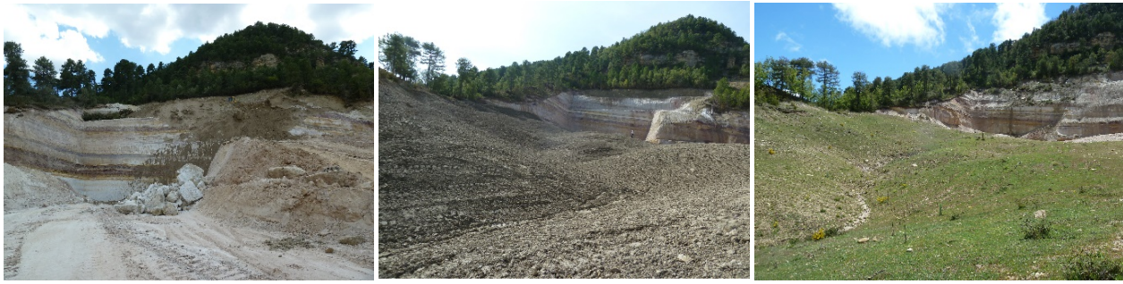
Figure 1 Geomorphic rehabilitation of a sector of El Machorro kaolin mine (Poveda de La Sierra, Guadalajara, Spain). Left, before rehabilitation (August 2012); centre, after landform regrading and soil replacement (October 2012); right, first stages of vegetation re-establishment (May 2014). Photos by José F. Martín
