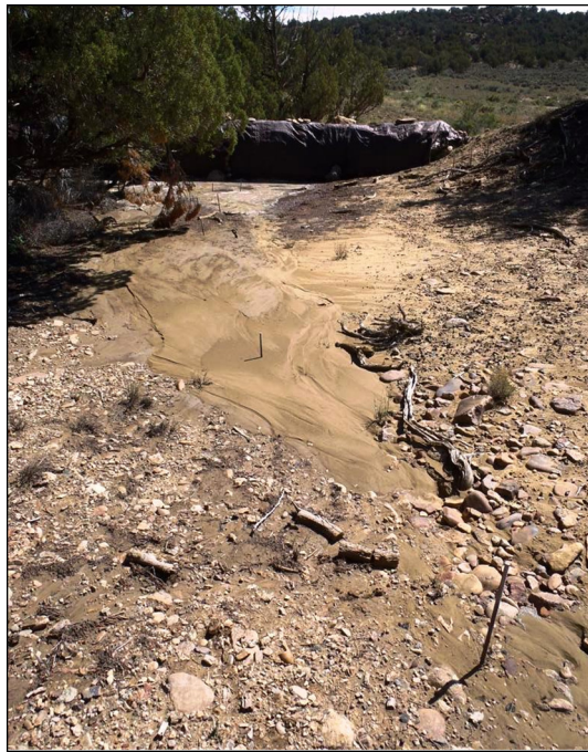
Fig. 12. View downstream to the N7 temporary sediment dam after the first sediment event.
