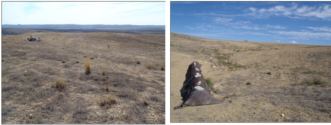
Fig. 9. MV5 subwatershed site. Fluvial geomorphic design with topdressing and poor to moderate vegetation establishment.
