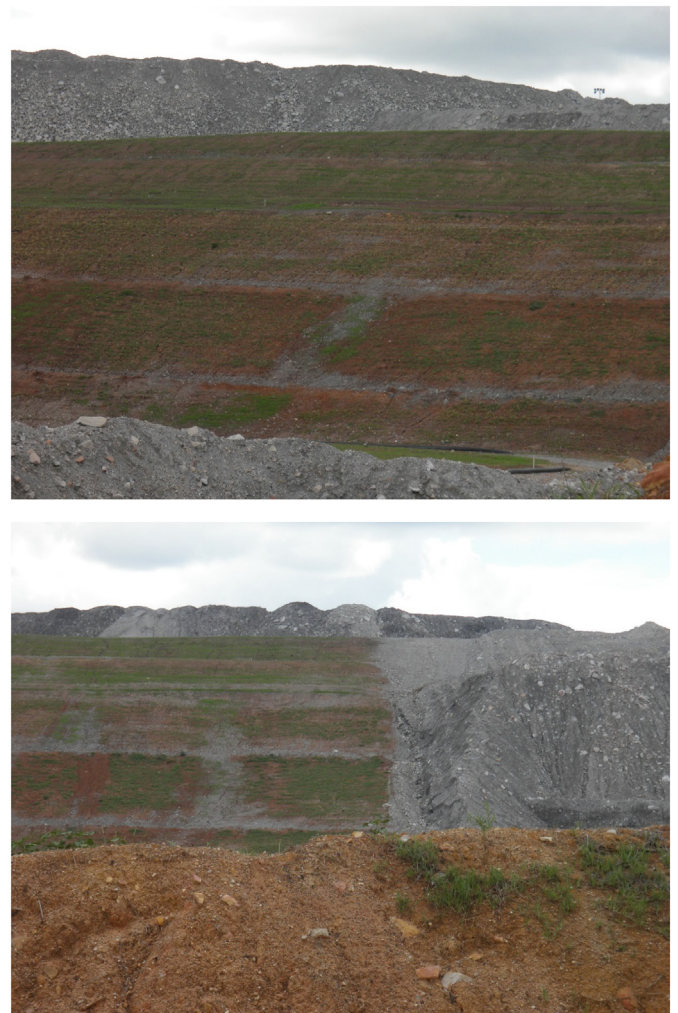
Fig. 7. A reconstructed landscape with benches and contour banks and initial revegetation. Rills and gullies can be observed (top). A partially rehabilitated hillslope with benches and contour banks displaying the underlying material and initial dump shape (bottom).
