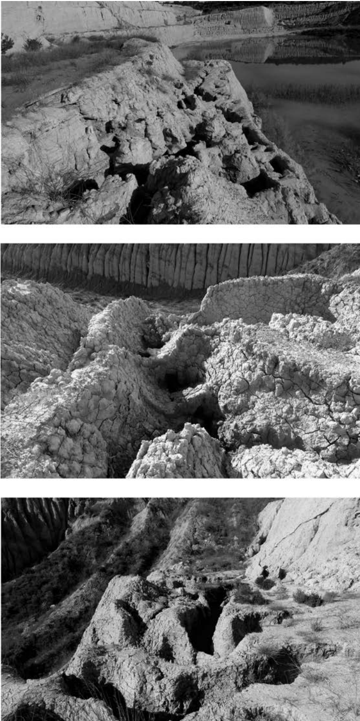
Figure 2. Tunnel erosion, piping, at benches of highwall terraces, at the Pastor I quarry.
