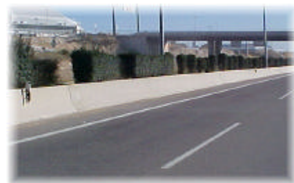
Barrera New Jersey "in situ"
